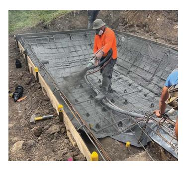
CONCRETE LINE PUMPING uses flexible hoses that can be manoeuvred to place concrete in a specific location. They are ideal for tight or hard-to-reach places, such as around buildings, tight alleyways, or difficult access locations. Line pumps are highly effective in both commercial and residential projects or where equipment and materials are limited.
