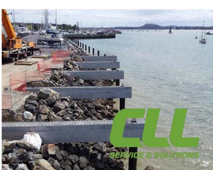
**Marine piling:** CLL/Oxcon CLL installed a total of 871 lineal metres of 610mm diameter tube piles - all within the CMA. The piles were initially spliced into 18m sections, driven, then spliced and re-driven as needed to achieve to the required set. A drop hammer, a 120-tonne crawler crane, and a 50-tonne hydraulic crawler support crane were used to drive the piles up to 35m into the existing East Coast Bays Formation (ECBF) below.
